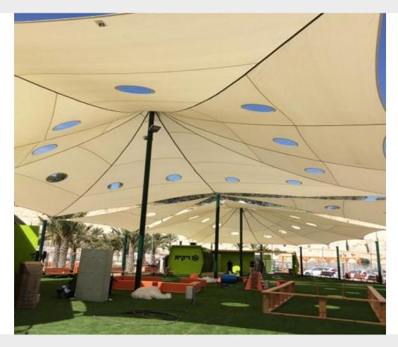
Like many outdoor structures, over time shade fabric can appear to be very dirty. The GALE Pacific range of shadecloth products are manufactured from High Density Polyethylene or HDPE. This material is quite inert to dirt, moisture and some chemicals. This is great, because dirt doesn't stick to the individual yarns in the fabric - additionally, HDPE wont rot like canvas and similar products.
